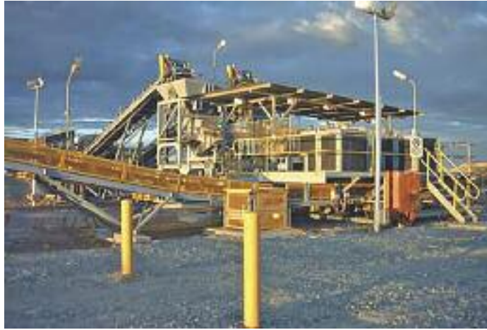
Applied Sorting installation at Leinster (nickel, Western Australia)
